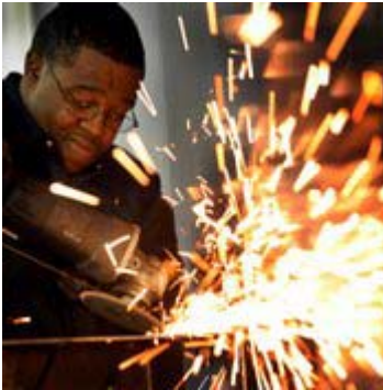
Jamey Williams of Albany grinds a steel door at Metal Supermarkets in Guilderland.
